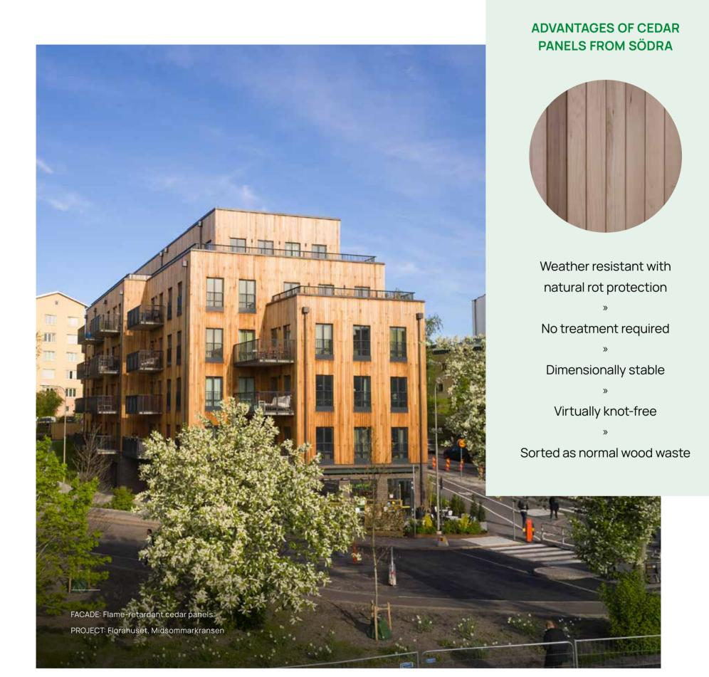
Södra's cedar is only offered in the highest quality, WRC Clear #2. This wood is ideal for exterior cladding and for various types of construction work.
